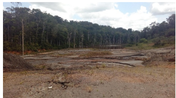
Figure 15. West Waste Storage Facility southeast creek entry point inundated by Main Pit runoff. Natural creek or creek bank no longer exists.
